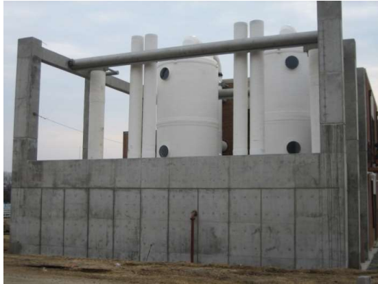
Picture #1: Richmond Treatment Plant, NRP-3 Project - Richmond Virginia
