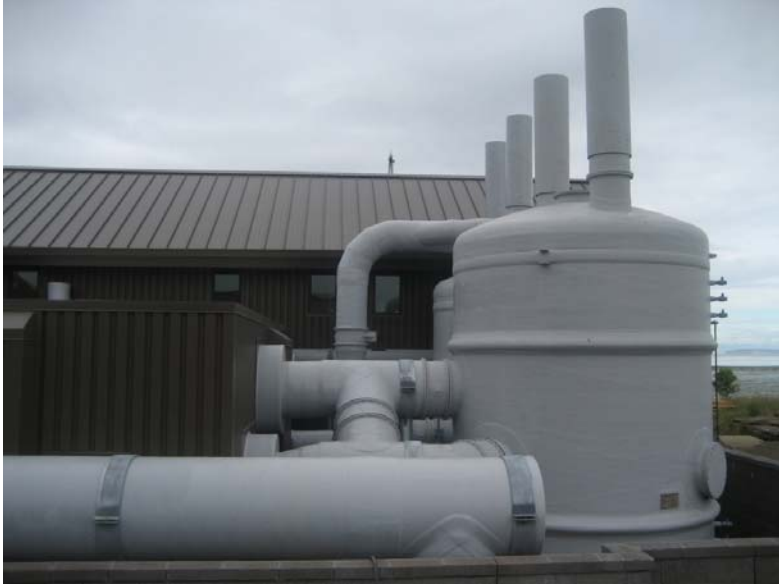
Picture #4: Blaine Lighthouse Point Water Reclamation Facility. Blaine, Washington
