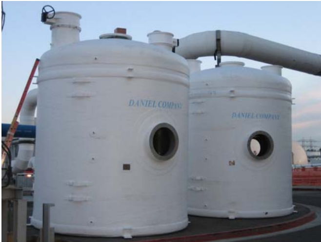
Picture #1: Hyperion Treatment Plant. Los Angeles, CA
