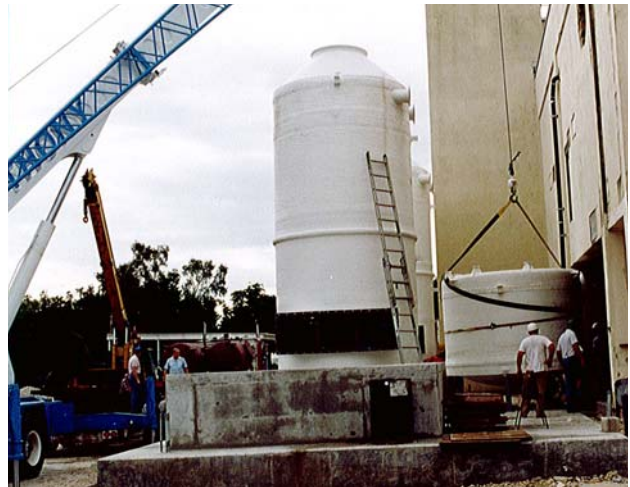
Photo #14: City of Hollywood, FL
